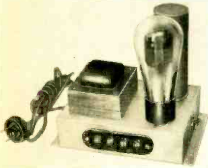
Above—a new and extremely compact power supply unit employing an 80 type tube and intended for use with short-wave A.C. receivers; diagram appears below. (No. 107.)
